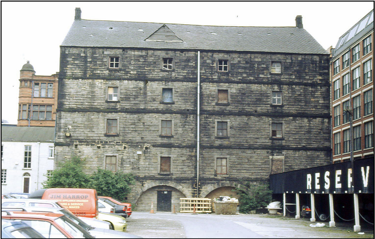
Above: Rochdale Canal: Ducie Street warehouse, Manchester (1998)
