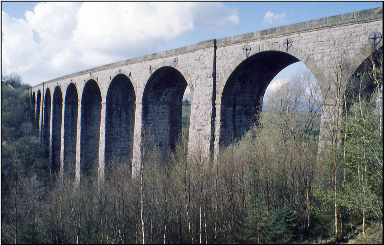
Above: Midland Railway, Settle & Carlisle Extension: Smardale Viaduct
