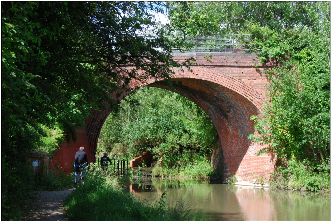
Wilts & Berks Canal: Skew Bridge, Swindon (former Midland & South Western Junction Railway)
